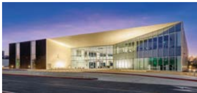
New Student Services Building
